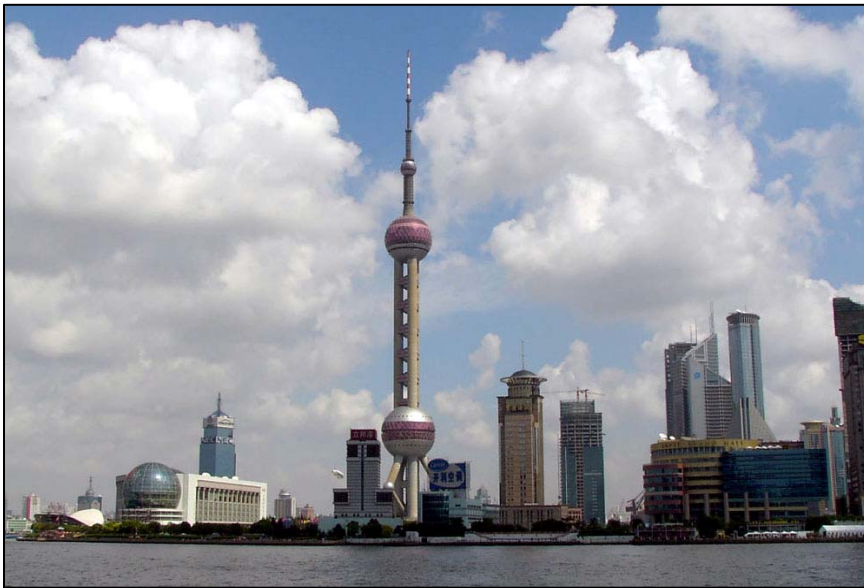
The Oriental Pearl Telecommunications Tower in Pudong, the east side of the Huang Pu River. It is the tallest building in Asia, with a convention centre alongside (the globe). Close by, a Japanese developer is erecting what will be the tallest skyscraper in the world.
