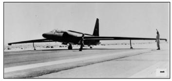
Then two of the crew push up the heavy wing, allowing a third crew member to install a pogo on the other side.
